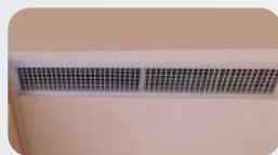
Front air flow, back air intake
