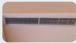
Front air flow, back air intake
